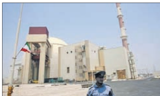
A security official stands in front of the Bushehr nuclear reactor, 1,200 km (746 miles) south of Teheran, on 21 Aug, 2010.—REUTERS
