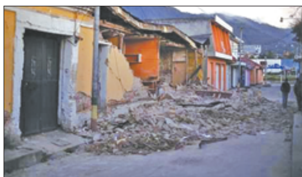
Two men walk past damaged houses after a 7.4-magnitude earthquake struck on Wednesday on the streets of San Marcos, in the San Marcos region, about 250 km (155 miles) south of Guatemala City, on 8 Nov, 2012.—REUTERS
