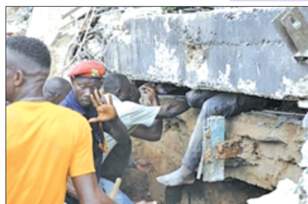
Rescue workers look for survivors from the debris of a collapsed building rented by Melcom Ltd, which runs Ghana's largest chain of retail department stores, in Accra on 7 Nov, 2012. —REUTERS
