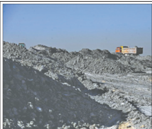
Trucks transport cinder in Shuozhou, north China's Shanxi Province, 31 Oct, 2012. As a city relying on coal power, Shuozhou has three major thermal power plants in its Shentou District. The thermal power plants emit some three million tons of coal ash each year. The pulverized fuel ash reclamation area, which used to be farmlands, is now covered with 120 million tons of coal ashes and becomes a huge pollution source.
