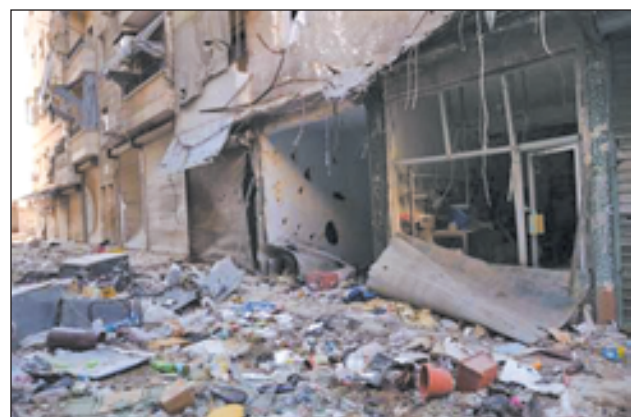
Damaged buildings are pictured in the Qastal al-Harami area, in Aleppo city on 3 Nov, 2012, after clashes between Free Syrian Army fighters and forces loyal to Syria's President Bashar al-Assad.—REUTERS
