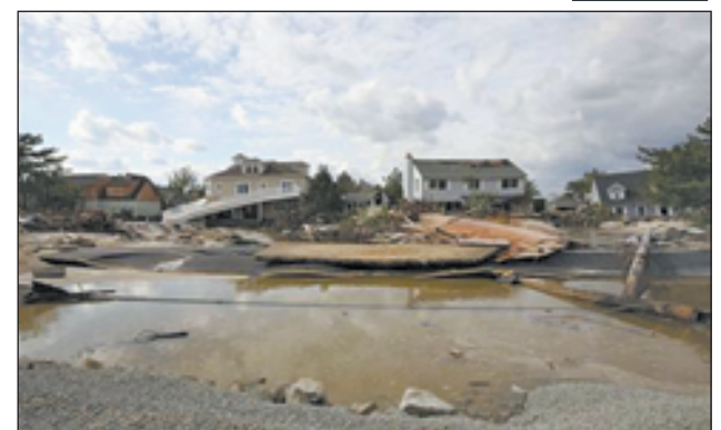
Hurricane Sandy damaged areas are seen along Rt 35 in Bayhead, New Jersey, on 2 Nov, 2012 in this handout image courtesy of the governor's office.
