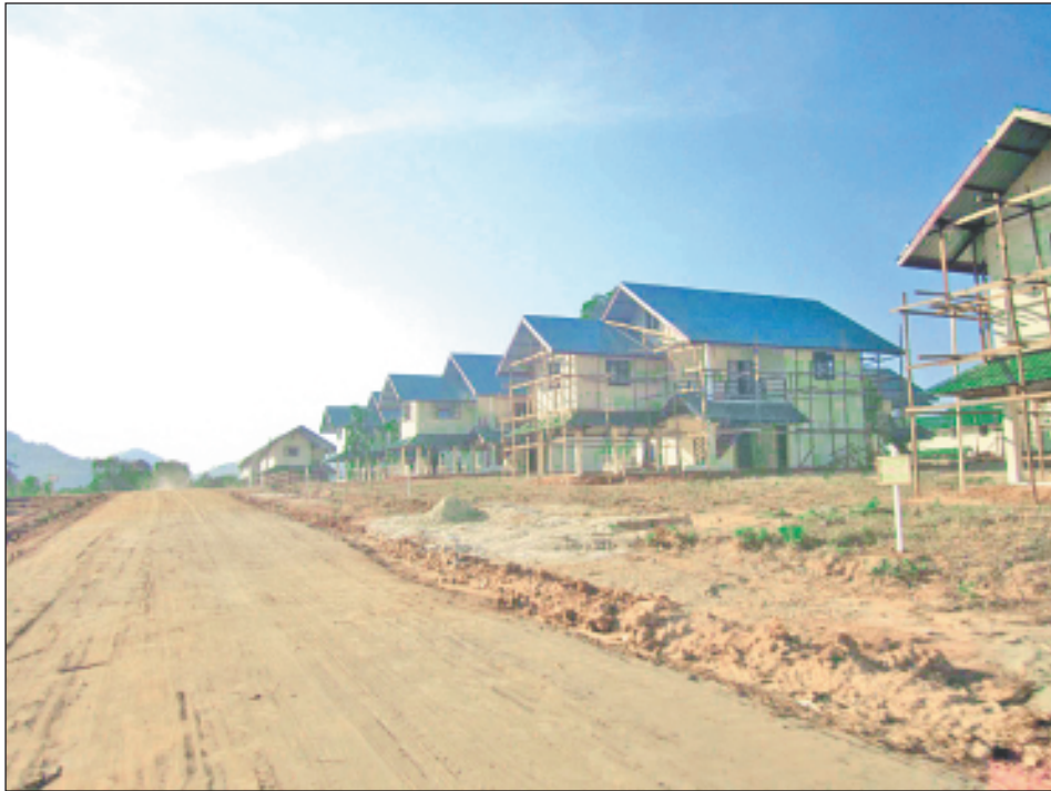
Photo shows progress of housing project.—MNA
