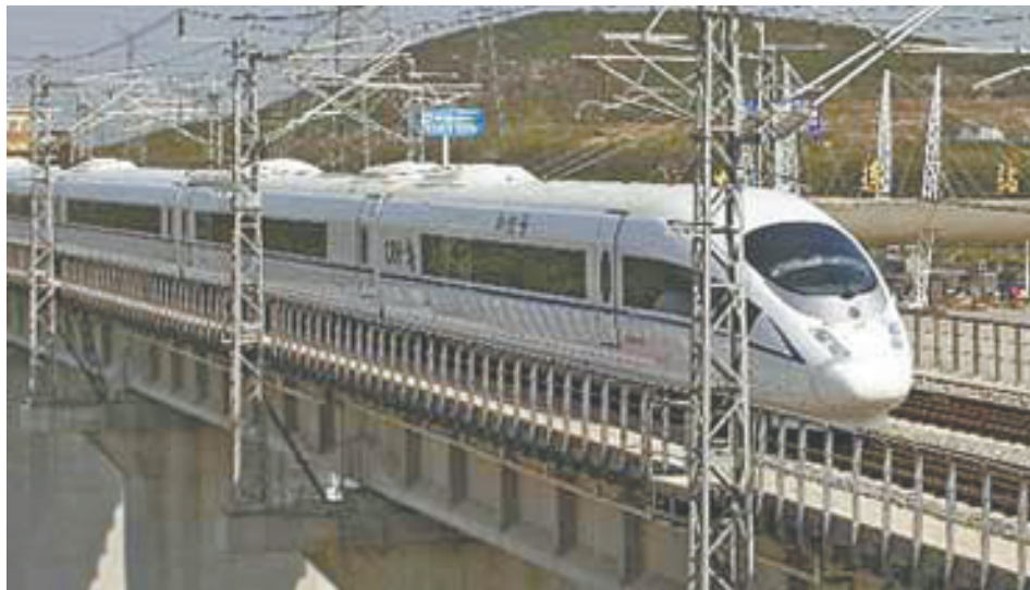
Work begins on major high-speed railway in western China.— XINHUA
