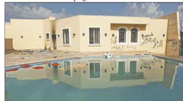
An exterior view of the US consulate, which was attacked and set on fire by gunmen in Benghazi, on 12 Sept, 2012.—REUTERS
