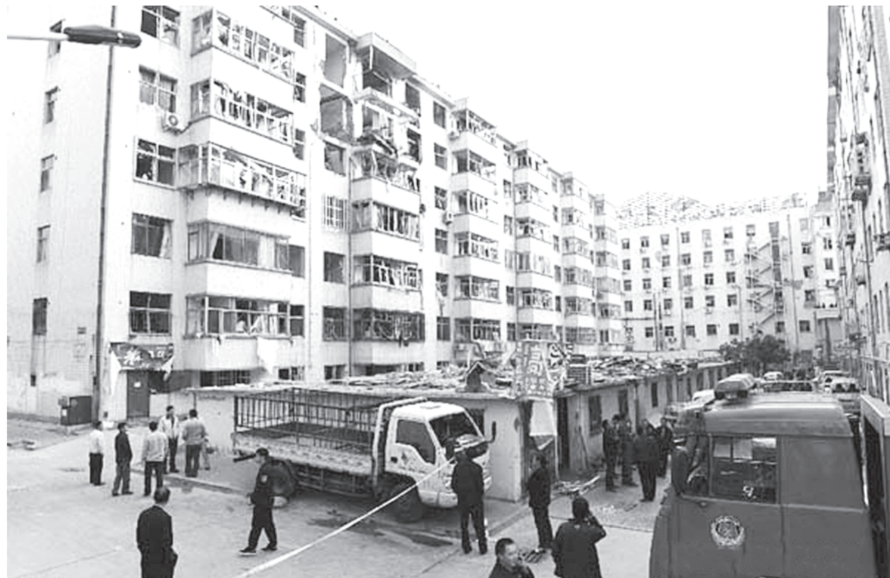
Photo taken on 15 Oct, 2012 shows the damaged building after an explosion in Weihai, east China's Shandong Province. At least one person has been confirmed dead and four other missing after an explosion ripped through the residential building in Weihai on early Monday morning. The blast hit the building's sixth floor at around 1 am and subsequently caused a fire. In addition to the dead and missing, 10 people were injured. Among them, three sustained severe injuries, said rescuers. Preliminary investigation indicated the blast was caused by a gas leak.— XINHUA
