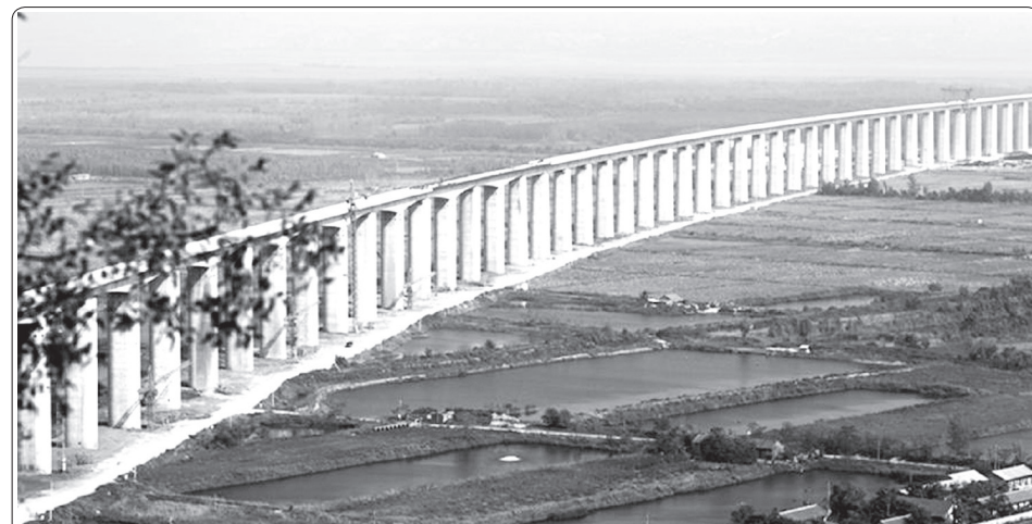
Photo taken on 9 Oct, 2012 shows the Jinshan Yellow River Bridge linking Yongji City of north China's Shanxi Province and Heyang County of northwest China's Shaanxi Province. The closure of the 9,969-metre-long bridge, which was a major project of the Datong-Xi'an passenger railway line, finished on Friday.— XINHUA
