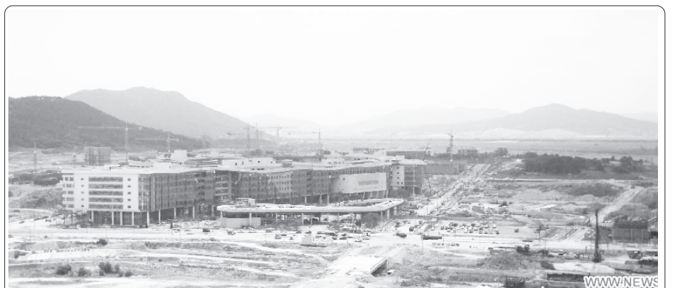
Photo taken on 3 July, 2012 shows a view of the government buildings under construction in Sejong City, 120 km south of Seoul, South Korea. More than 100 staff members of six departments of Prime Minister's Office started to move to Sejong City, the new administrative city, on 14 September. Sejong City will eventually house 36 government ministries and agencies by 2014. Its current population of 120,000 is projected to jump to 500,000 by 2030. — Xinhua
