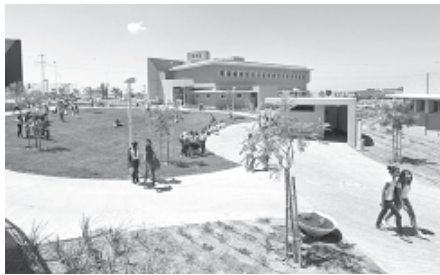
Israeli high-school students walk through the yard next to a new rocketproof school building, in Shaar Hanegev school, near the southern town of Sderot, Israel, on 27 Aug, 2012. The 27.5 million US Dollar structure features concrete walls, reinforced windows and a unique architectural plan all designed specifically to absorb rocket fire.—INTERNET
