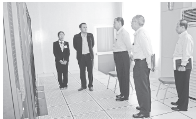
Union CPT Minister U Thein Tun looks around machine rooms at the main building of Yatanarpon Teleport. MNA
