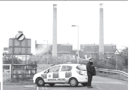
Smoke rises from Tilbury power station during a fire at the plant in Essex on 27 February, 2012. REUTERS
