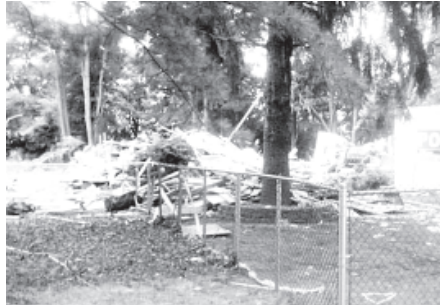
A pile of wood, plywood, drywall, insulation and other building material is all that remains after an apparent gas-related explosion leveled a house in Brentwood, NY, on 14 Aug, 2012.
