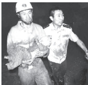
A firefighter rescues a child from an accident site after a road collapsed at Liaoyang Street of Harbin City, northeast China's Heilongjiang Province, on 14 Aug, 2012. XINHUA
