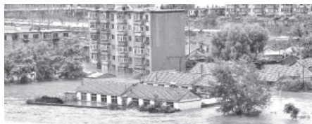
Buildings are inundated in flood water in Nanfen areas of Benxi, northeast China's Liaoning Province, on 4 Aug. 2012. Flooding triggered by torrential rain brought by Typhoon Damrey, the 10th typhoon of the year, disrupted services of three railways in Liaoning Province. Rescue is underway.
