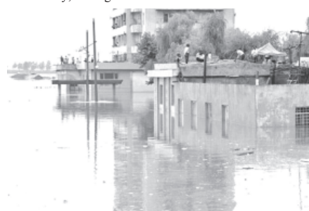
Flooded houses in Anju city in South Phongan Province. The Red Cross said on Thursday it had allocated almost $308,000 for victims of North Korea's floods and storms, after state media reported 119 deaths and major crop damage in the food-scarce nation. — INTERNET
