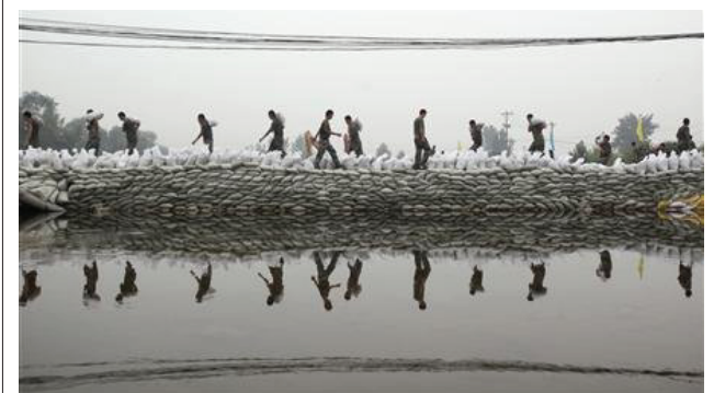
Chinese People's Liberation Army soldiers place sandbags to block a breaching dyke after heavy rainfalls hit the Fangshan district of Beijing, on 25 July, 2012.
