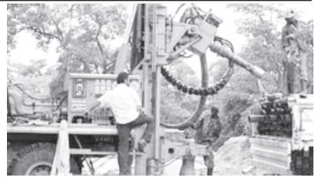
Test drilling on the new aquifer.— INTERNET
