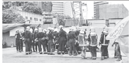
Singaporean rescuers gather outside the Downtown Line (DTL) Bugis Station subway construction site in Singapore on 18 July, 2012.—INTERNET
