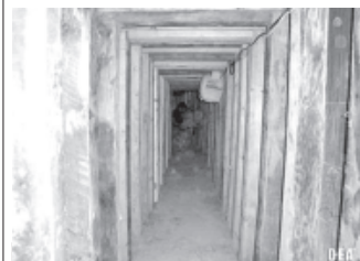
The interior of a cross border tunnel is pictured in this undated handout photo taken by the DEA in San Luis, Arizona.
