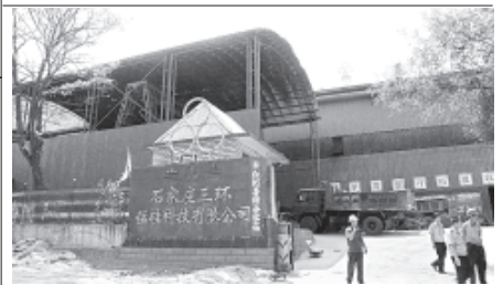
Photo taken on 3 July, 2012 shows the Xiaojue Branch Plant of Shijiazhuang Sanhuan-Smelting Co Ltd where an accident of slag water leakage occurred, in Xiaojue Township of Pingshan County, north China's Hebei Province. Six people were suffocated to death when slag water leaked in this plant and mixed with rainwater on Tuesday.—XINHUA
