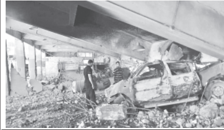
Palestinian security members inspect a damaged car at Hamas security building which was targeted in Israeli air raid in Gaza City, on 23 June, 2012. Israel’s military raids continued in the Gaza Strip on Saturday. — XINHUA
