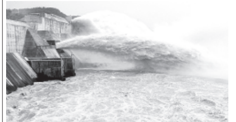
Water gushes out from the Xiaolangdi Reservoir on the Yellow River during a sand-washing operation in Mengjin County, central China's Henan Province, on 20 June, 2012. The Yellow River has been plagued by an increasing amount of mud and sand.—XINHUA
