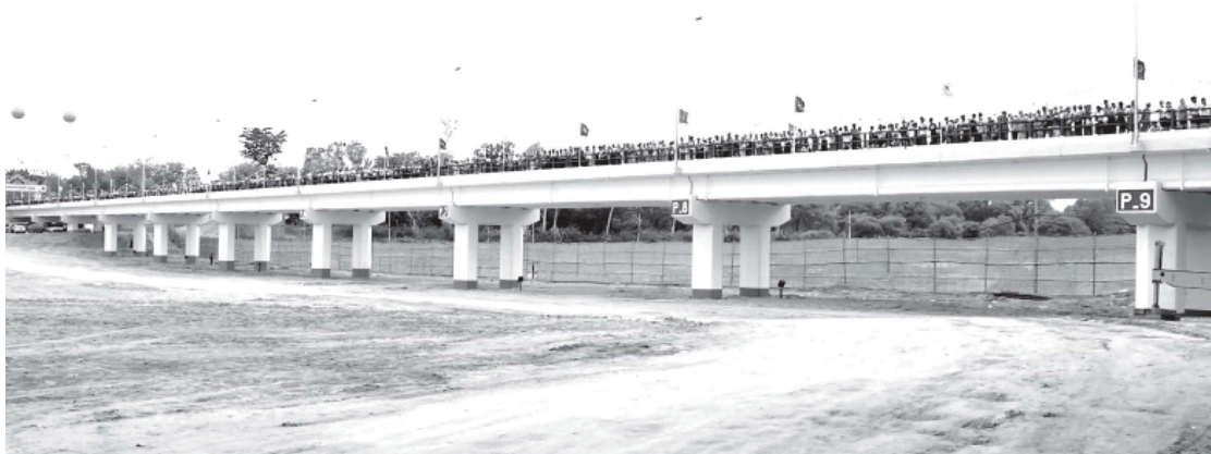
Shwechaung Bridge No. 1 on Pakokku-Monywa road in Pakokku Township.—MNA
