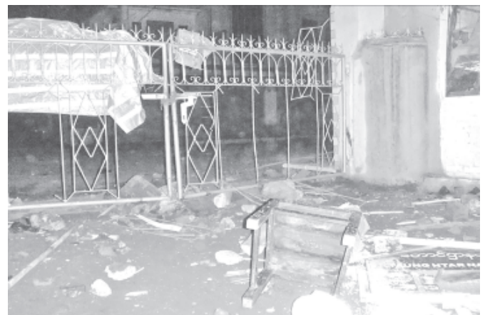
Damaged gate of police station.—MNA
