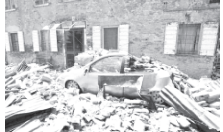
A car is covered in debris after the roof of a quake-damaged house collapsed in Cavezzo. A strong earthquake has rocked northeastern Italy, just days after another quake in the same region wrought death and destruction. — REUTERS
