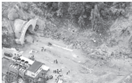
Photo from helicopter shows the site of an explosion that occurred at a tunnel construction site in Minamiuonuma, Niigata Prefecture, on 24 May, 2012. NHK
