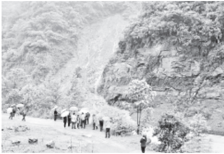
Photo taken on 22 May, 2012 shows the landslide site on the No 319 national highway beside the Wulingshan Tunnel in Chongqing, southwest China. The rainstorm-triggered landslide, which happened at around 11:00 am, resulted in an accumulation of more than 10,000 cubic metres of earth and stone and cut off traffic from Qianjiang District to Pengshui County in Chongqing, said Zhou Xinguo, deputy director of the district's transportation commission. —XINHUA
