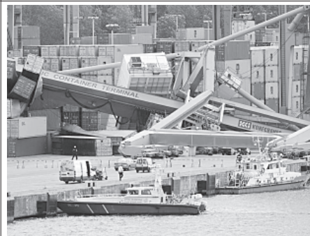
People look on after the gantry of the Baltic Container Terminal fell down onto shipping containers at the waterfront in Gdynia, Poland on 17 May, 2012. Three people were injured in the accident.—INTERNET
