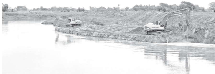
Silt from Bago River being dredged by machinery for proper flow of the river.—MNA
