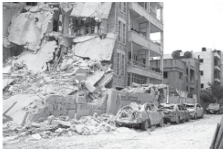
A view of the damage at the site where two bombs detonated near state buildings in the northern city of Idlib on 30 April, 2012.—REUTERS
