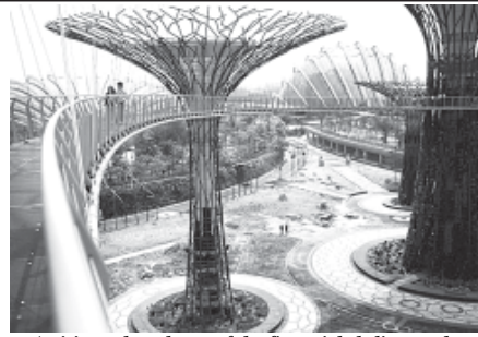
A visitor takes photos of the financial skyline on the 'OCBC Skyway' linking the Supertrees, ranging from 25-50 metres in height and serving as vertical gardens in the newly completed Gardens By The Bay just next to Singapore's busy financial district. INTERNET
