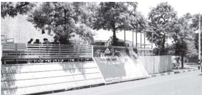
Sein Sabei Phu, Crystal (Tawwin Diamond House) is under construction.
