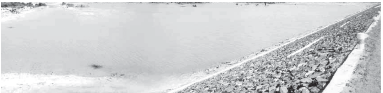
Photo shows Kyauksauk Dam.
