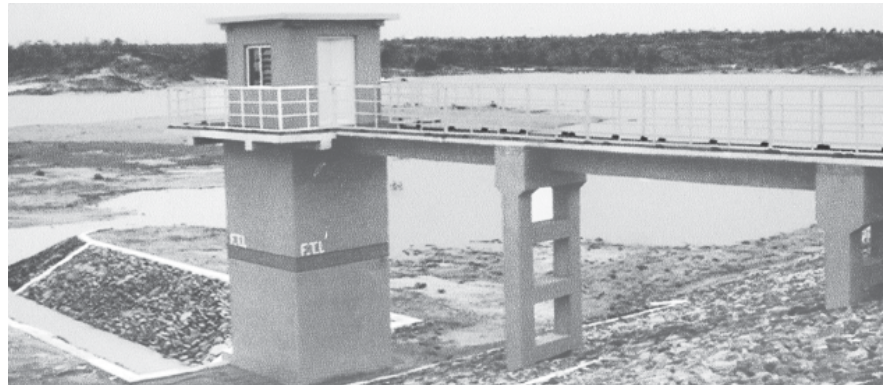
Control Tower of Ngachin Dam.
