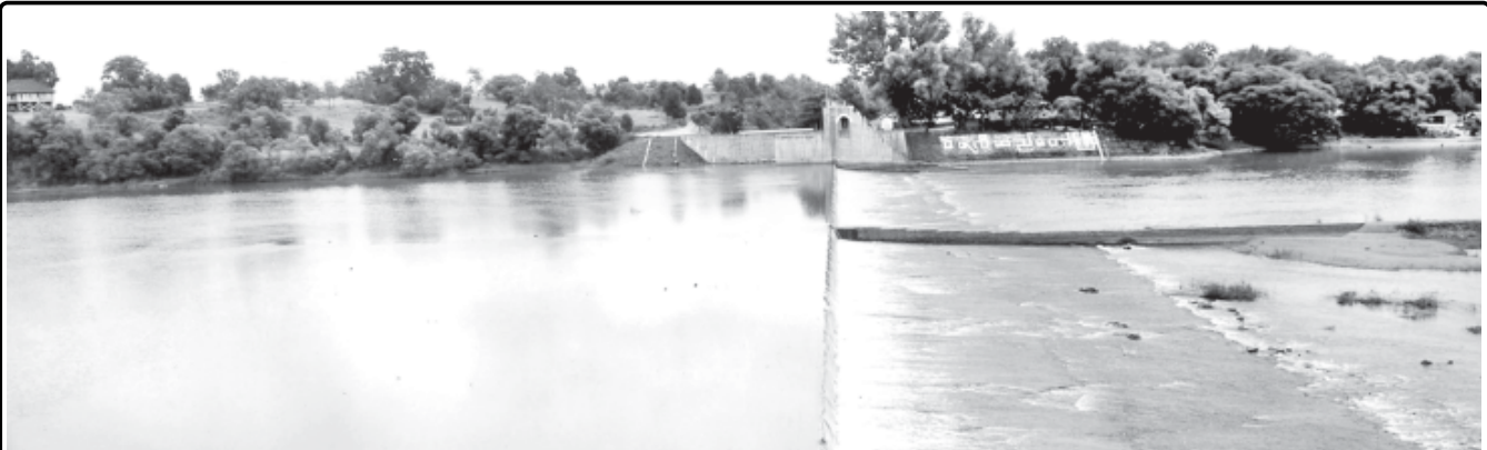
Mezali Diversion Weir supplying irrigation water to plantations in the region.
