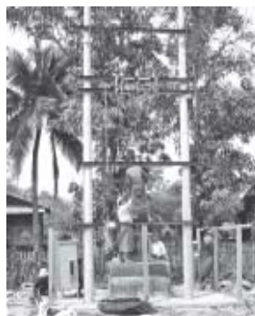
Electricians installing transformer in Mawlu region.
