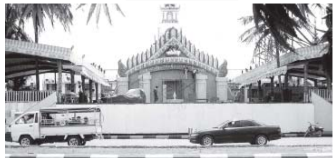
Photo shows progress of Mandalay Mayor's Water Throwing Pandal.
