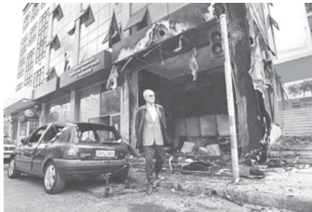
A man walks in front of a damaged Administrative Reform ministry building in Athens on 9 April, 2012.—REUTERS
