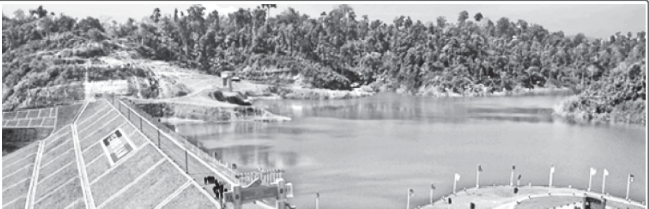
Yenwe Dam in Kyaukdaga Township, Bago Region.
