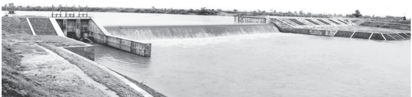
Baida Diversion Weir in DaikU Township, Bago Region.
