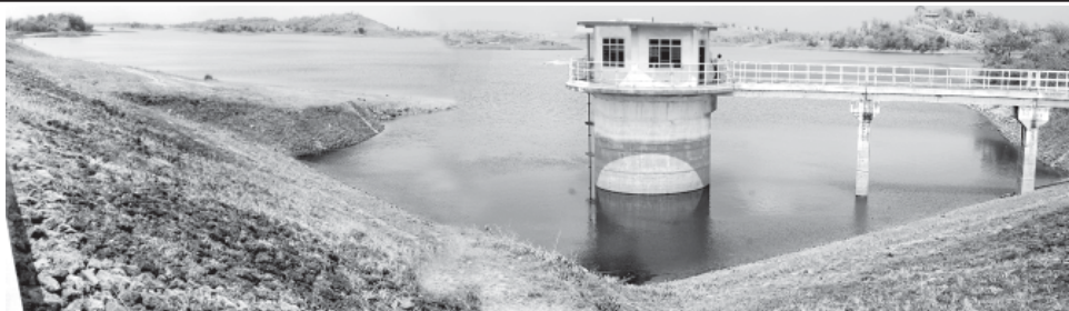
Wegyi Dam supplying irrigation water to farmlands in Paungde Township, Bago Region (West).
