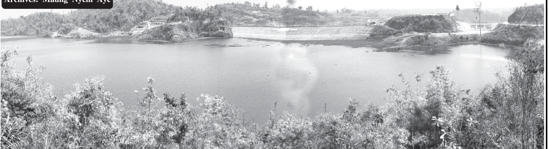
Khabaung Dam in Ottwin Township, Bago Region, stored with water.
