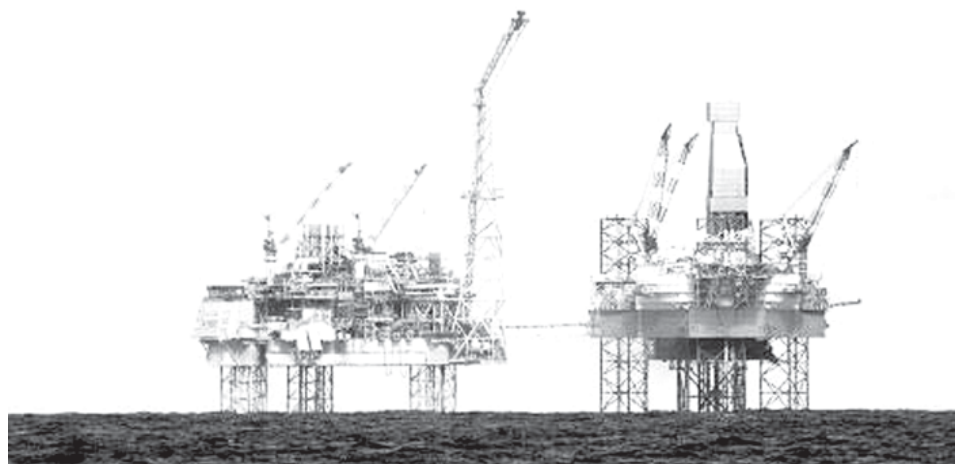
French energy giant Total's Elgin rig, 150 miles (240 kms) from Aberdeen. A team of experts spent four hours inspecting a wellhead that is spewing a cloud of potentially explosive gas on a North Sea platform operated by French energy giant Total, the company said on Thursday.— INTERNET
