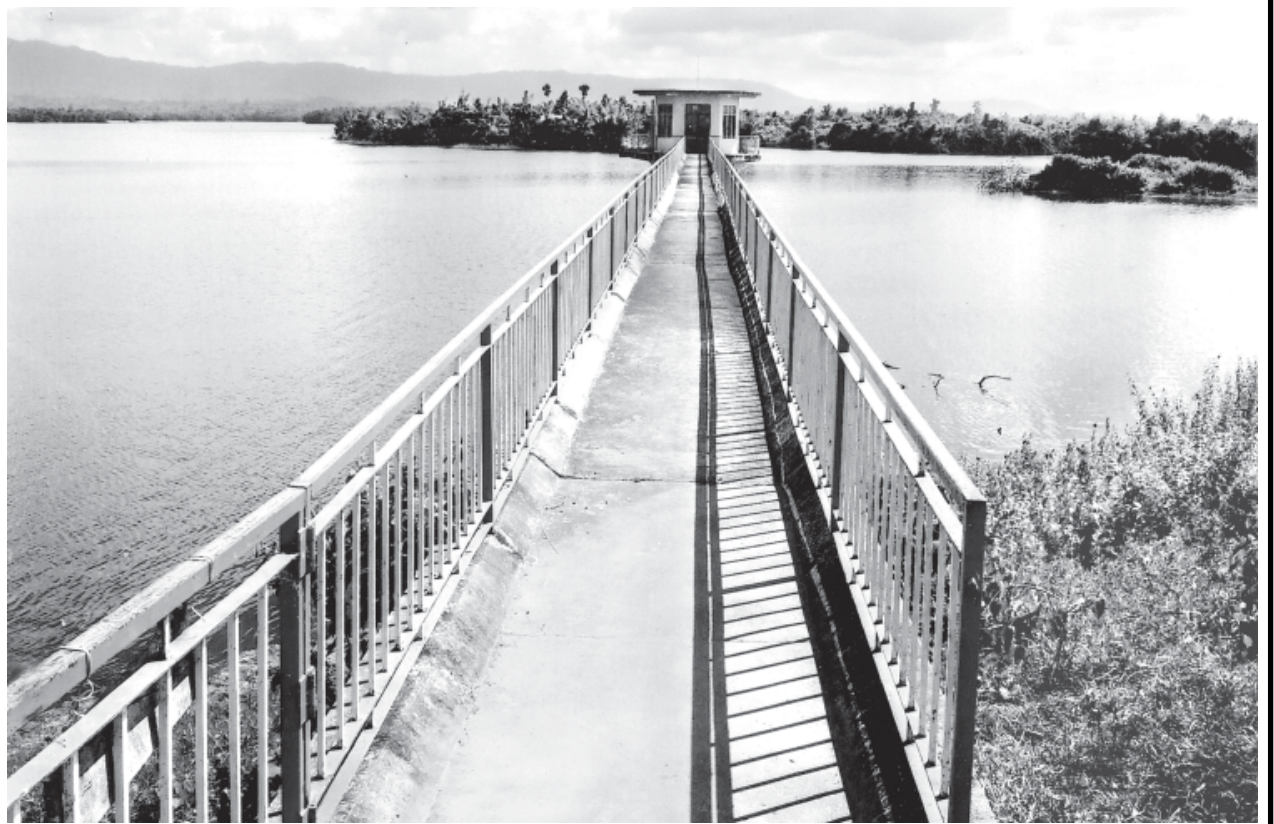
Bawbin Dam and Control Tower seen in supplying irrigation water to 30000 acres of farmlands in Bago Region.
