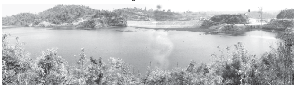
Khabaung Dam in Ottwin Township, Bago Region, stored with water.
