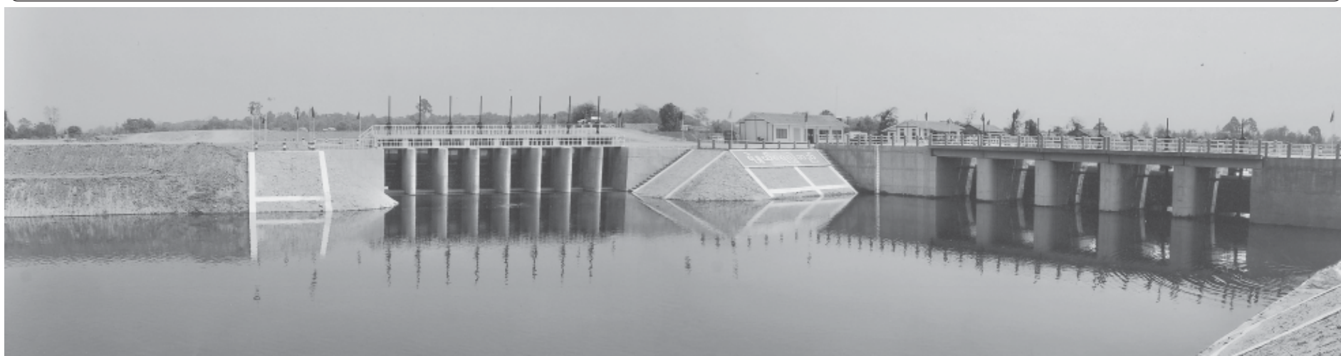
Sluice gate and valves of Yenwe diversion weir.
