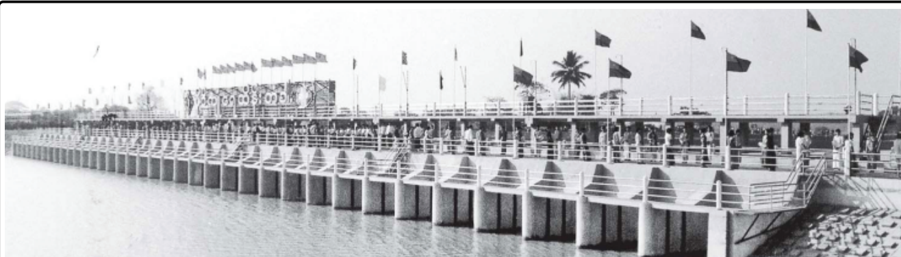
Paingkyon Sluice Gate supplying irrigation water to over 30,000 acres of farmlands in Kawa Township, Bago Region.
