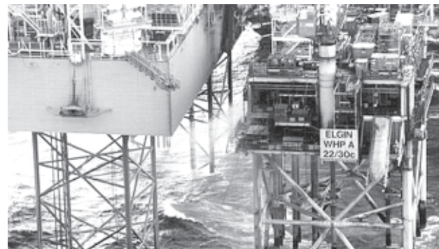
The leak at Elgin platform, 150 miles off Aberdeen, had been ongoing since Sunday. INTERNET
