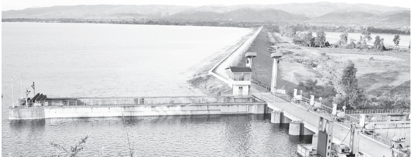
Moby Dam near Moby village in Pekhoh Township of Shan State (South) generates electricity and supplies irrigation water.
