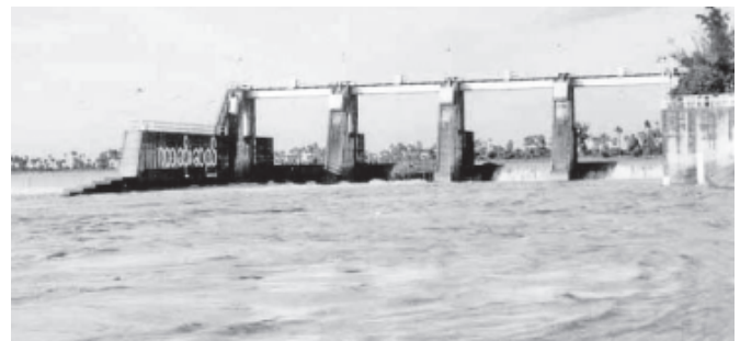
Karboe Dam supplies potable and irrigation water to local national people in Kachin State.
