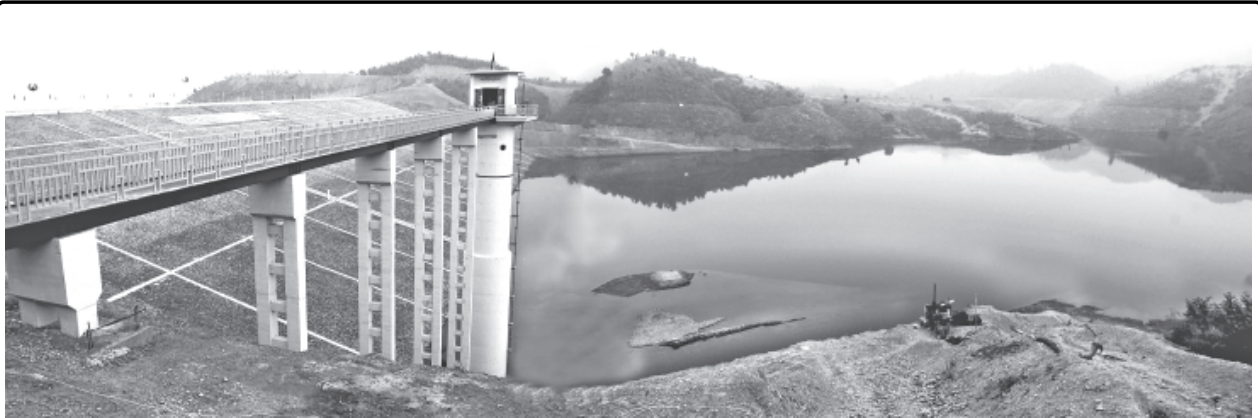
Zeechaung Dam for supply of irrigation water in Kyauktaw Township.
