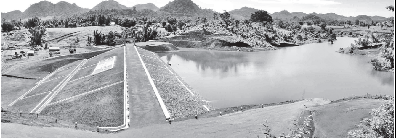
Nantkyan Reservoir in Lashio Township of Shan State (North) distributing potable water and irrigation water to local national races people in the region.
