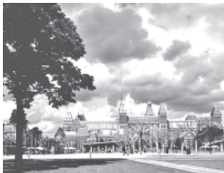
This file handout photo shows Amsterdam's Rijksmuseum. The museum is currently undergoing a major restoration ahead of a scheduled reopening in 2013.—INTERNET
