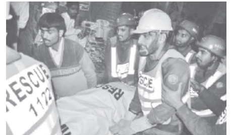
Pakistani rescuers transfer an injured man to a hospital at the collapsed building site in Multan, Pakistan, on 23 March, 2012. One woman was killed and 12 others including 6 children were injured when a three-storey building collapsed in Pakistan's central city of Multan on Friday night, said rescue workers and hospital sources.
