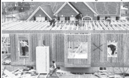
Workers build a new house in Alexandria, Virginia on 16 Feb, 2012.—REUTERS
