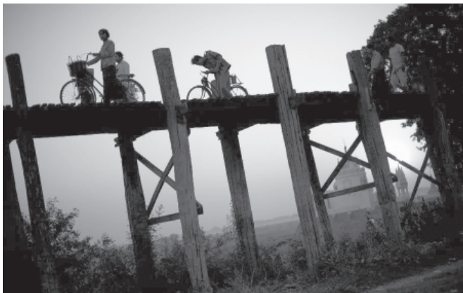
U Pein Bridge spans over Taungthaman Lake.—XINHUA
