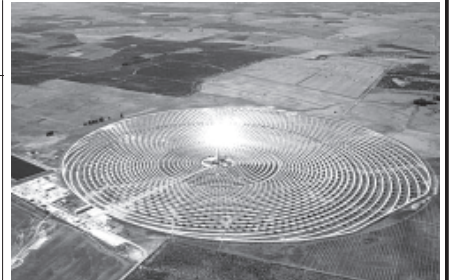
The Torresol Energy Gemasolar plant in Fuentes de Andalucía near Seville.—INTERNET
