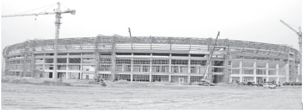
Progress in construction of Zabuthiri Stadium in Nay Pyi Taw.—MNA
