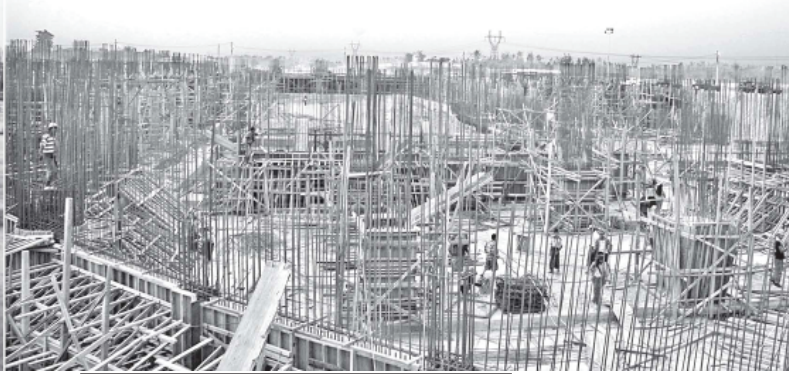
Vice-President Thiha Thura U Tin Aung Myint Oo inspects construction of Zabuthiri Stadium. MNA
