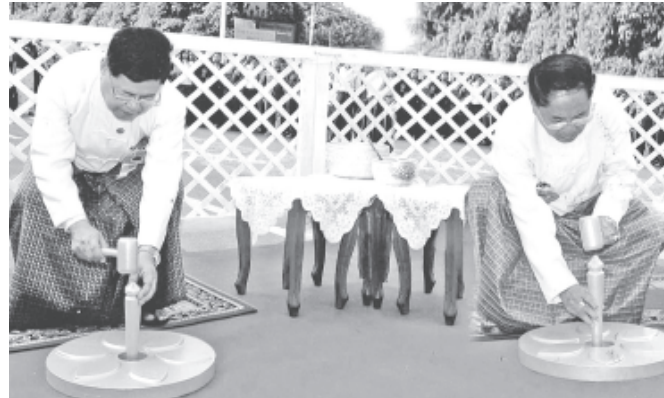
Union Minister for Industry U Soe Thein and Region Chief Minister U Myint Swe drive stakes for construction of an overpass at Hledan Junction in Kamayut Township.—MNA
