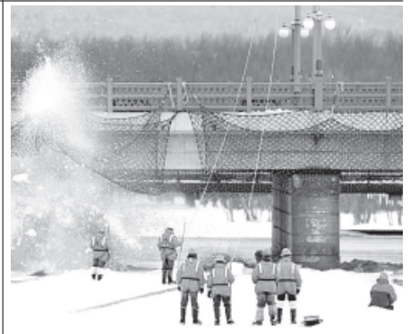
Municipal workers conduct their annual ice blasting work, using explosive charges and excavating equipment, to break up the ice and alleviate possible spring flooding on the Rideau River on 3 March, 2012 in Ottawa, Canada.—XINHUA
