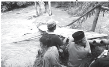
Residents examining a bamboo bridge that collapsed into the Cihideung River on Sunday in Cibanteng, Bogor. Antara Photo/Jafkhairi Residents examining a bamboo bridge that collapsed into the Cihideung River on Sunday in Cibanteng, Bogor.—INTERNET
