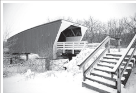
The Cedar Covered Bridge is covered with snow in Winterset, Iowa, the United States, on 13 Feb, 2012. More than a decade after the movie "The Bridges of Madison County" was released, thousands of people still travel to Winterset each year to trace the steps where Clint Eastwood and Meryl Streep immortalized the area's covered bridges. —XINHUA
